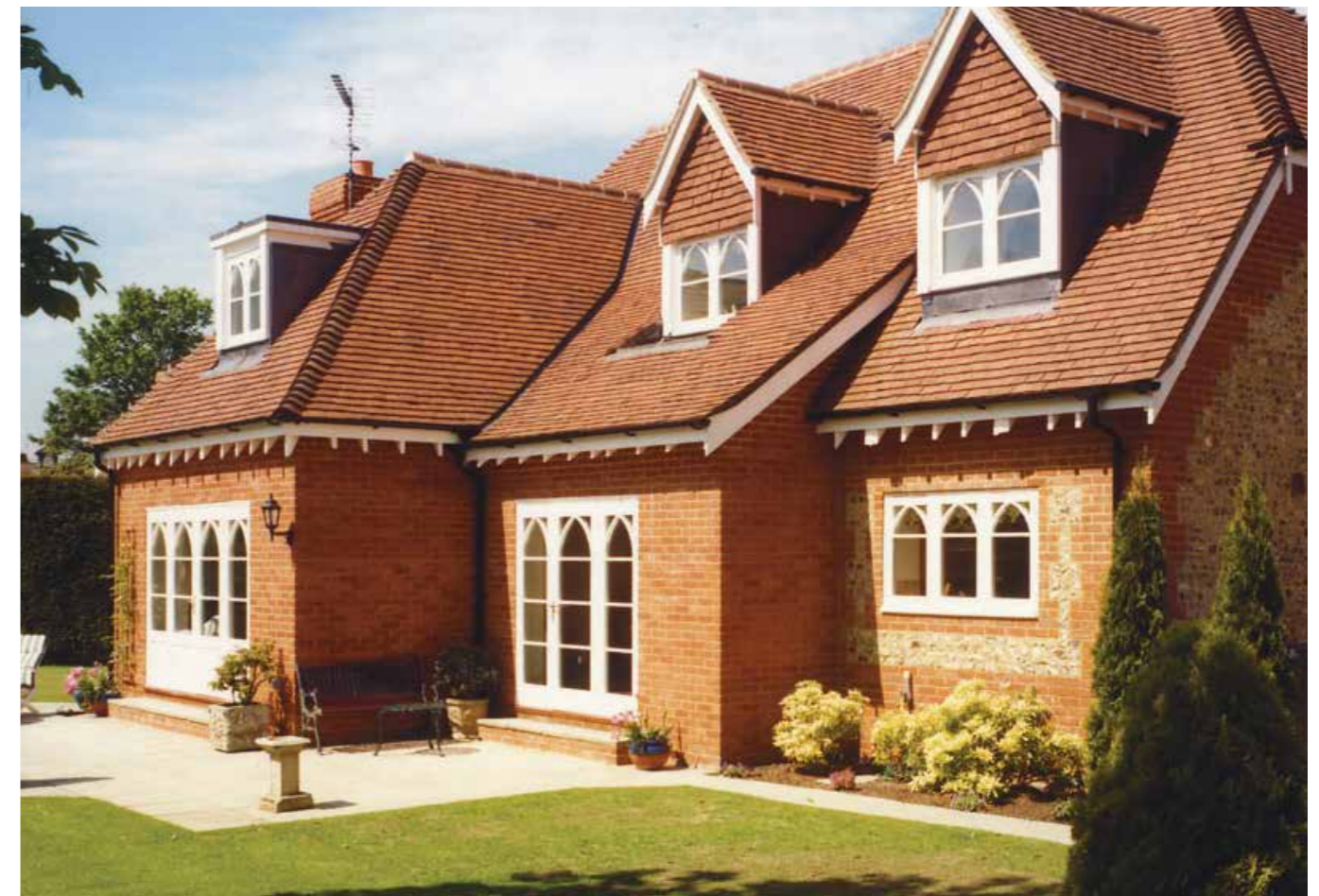
BEWLEY HOMES SOUTH WARNBOROUGH
