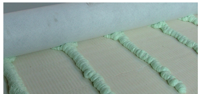
A bonded membrane incorporating HARDROCK® Multi-Fix (DD)
