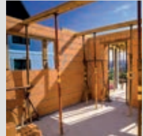
RAISING LOAD-BEARING WALLS
