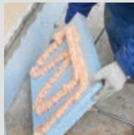
FILLING GAPS BETWEEN INSULATION BOARDS
