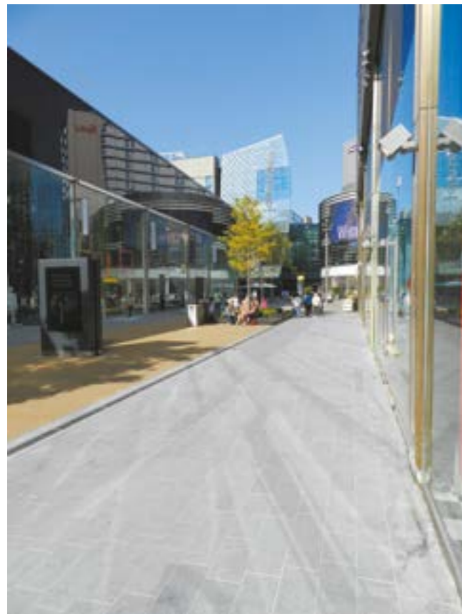
Podium Deck Waterproofing - Westfield Olympic Park, London
