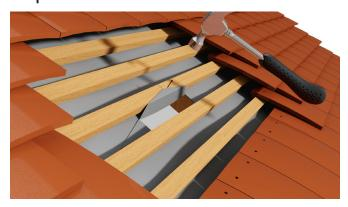
The top and side underlay triangular shapes should be folded outward and underneath the ventilator. The top triangle should be tacked to the batten above.
