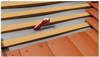
Once the position of the ventilator has been determined, mark and cut the underlay in a V-shape to the size shown below.
