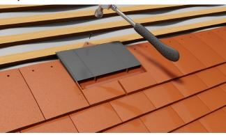
Position the ventilator with the spigot through the underlay cut and nail the ventilator to the batten through the hole in the top flange. Step 5
