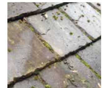
Greys Artstone GRC Slate (Glassfibre Reinforced Concrete)
