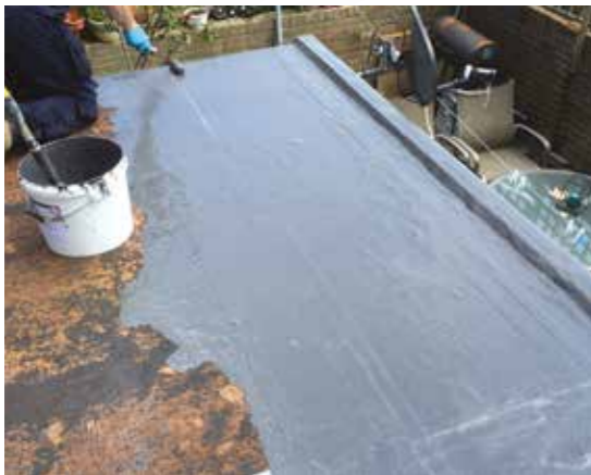
Apply a base coat of FIX-R Liquid Roofing
