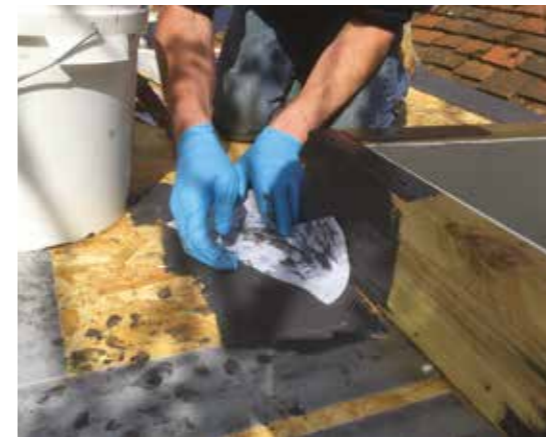
Detailing to roof light reinforced with fabric
