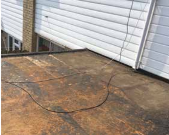
Surface before application
