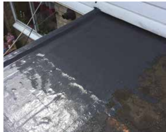
Apply FIX-R Fabric to reinforce
